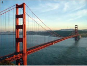
Cable-girder system (suspension bridge)
