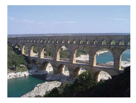
included them in buildings, bridges, and aqueducts. One of the most famous examples is the Pont du Gard, shown in Fig. 6.4; a bridge/aqueduct over the river Gard built in 19 BC. Some of the stones weigh up to 6 ton.
