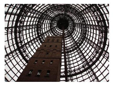
Fig. 2.13 Three-dimensional truss roof system
